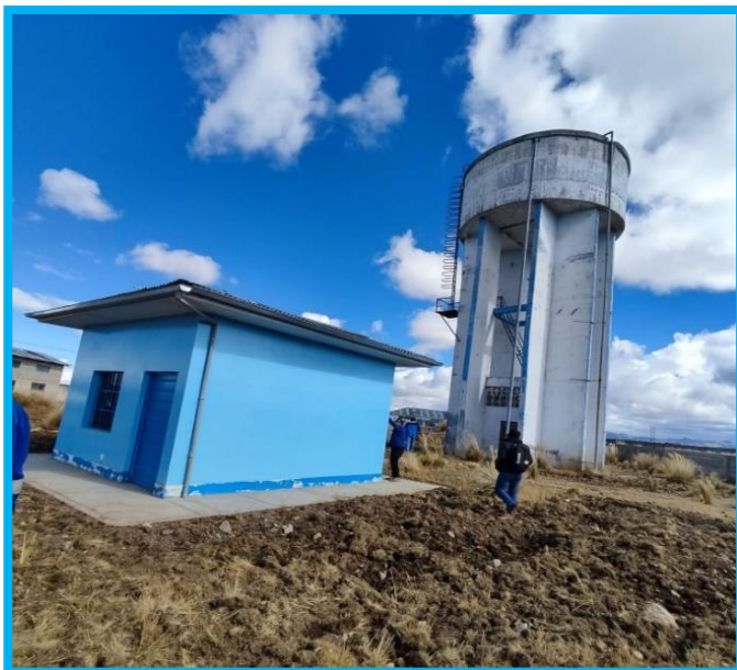
RESERVORIO TUPAC AMARU
